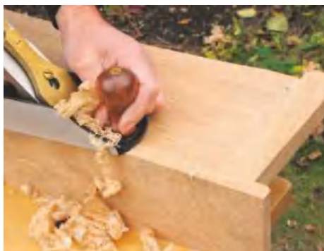
STEP 15. Trim the upper shelf edge flush at the rear of the coat rack with a smoothing plane
